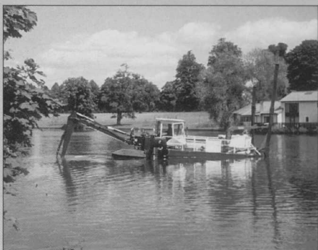
The amphibious Watermaster dredger 'walked' into the lake to clear it of weeds and reeds before dredging it
