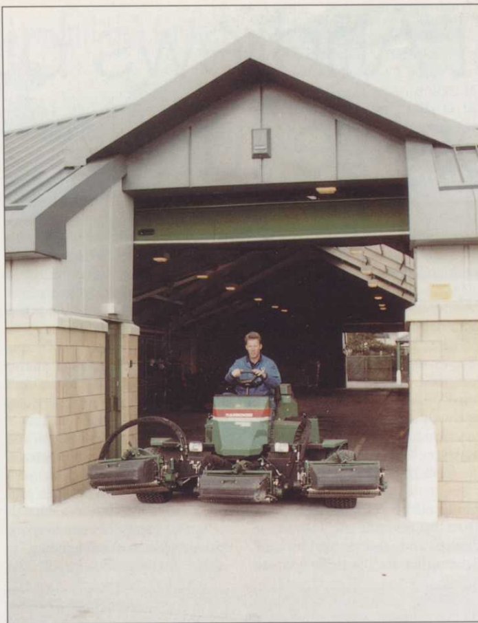
The main doors are set into the roof dormer-fashion to maintain a low eaves and building height in keeping with local architecture
