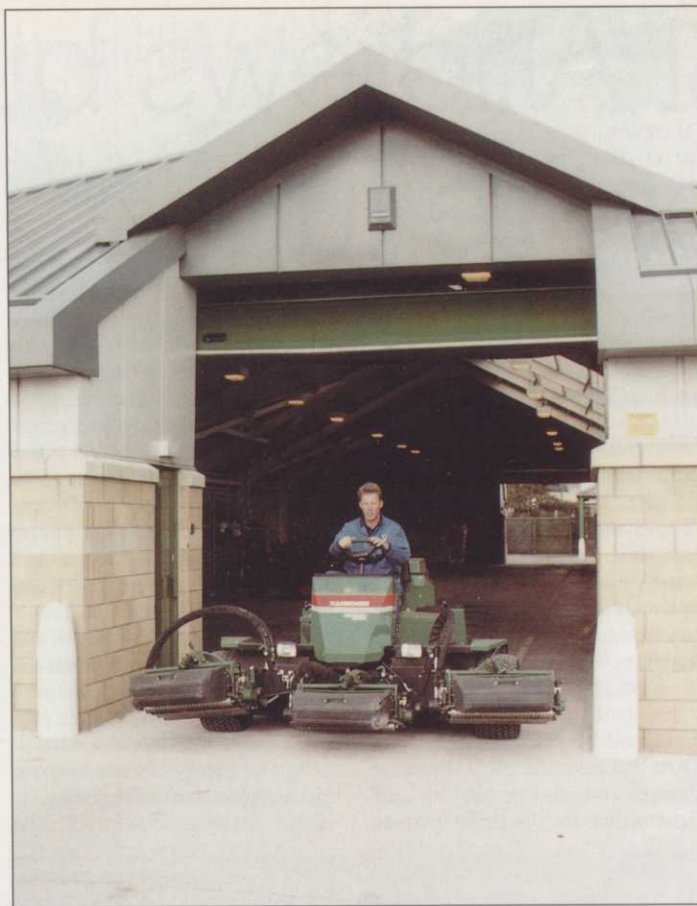
The main doors are set into the roof dormer-fashion to maintain a low eaves and building height in keeping with local architecture
