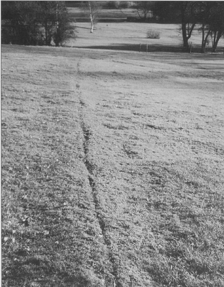
Now you can hardly see the join: After the work the heave has gone and the fairway is returning to normal
