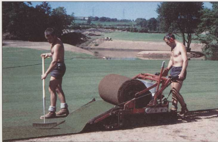
Installing big rolls
