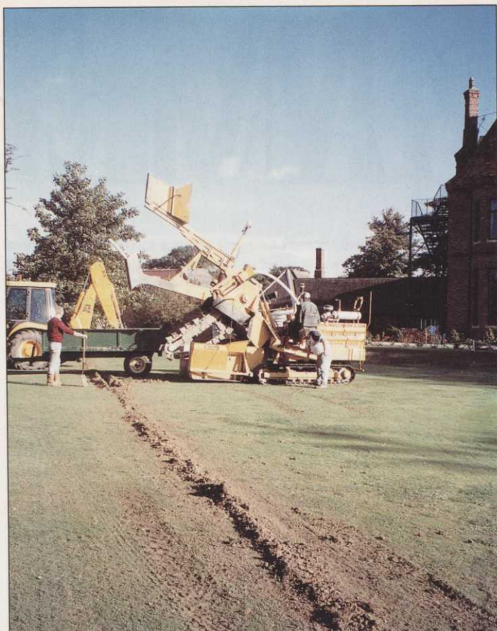
Drainage work being carried out at BIGGA's HQ, Aldwark Manor
