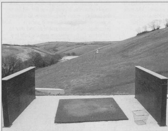
The driving range, with a dangerous slope for maintenance
