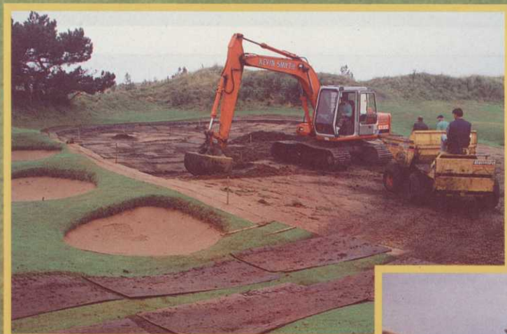
Main picture: the 5th green, with rootzone layer Left: the stage before – digging it up Below: how it looks today, with the green finished and bunkers remodelled
