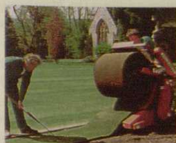
STANDARD SIZE OR BIG ROLLS. EXPERT LAYING SERVICE AVAILABLE.
