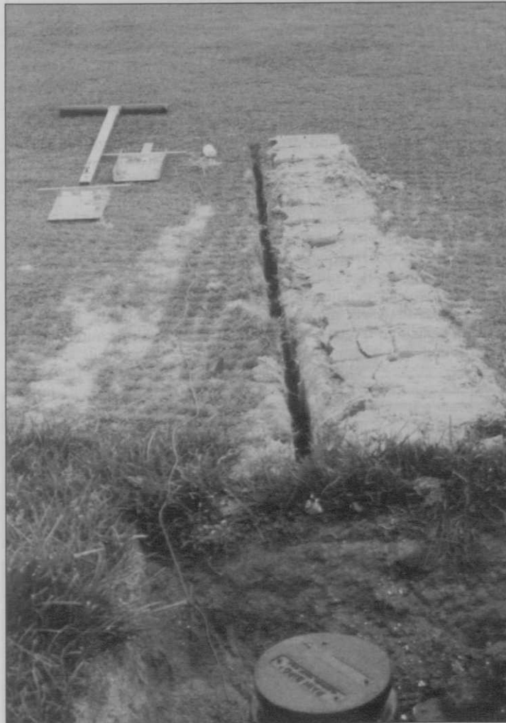
Installed: a moisture core in the green
