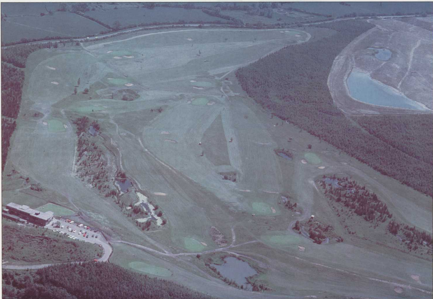
An overall view should be taken on upgrading work, particularly with drainage system improvement
