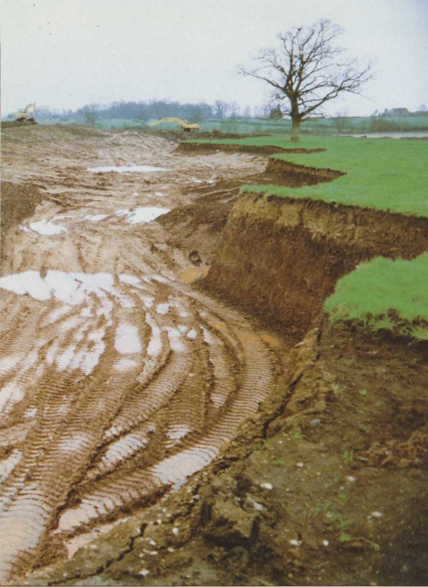
Pond under construction: clay seals are not necessarily easy to form. Vertical faces require special treatment
