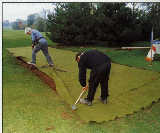
Erosion problems at Sceptoft Golf Club. The pictures show the appalling state of a high wear area and VHA carpet being installed below the surface, through which natural grass will grow. Photographs courtesy of Notts Turf
