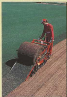
Fast turf laying: Big Roll
