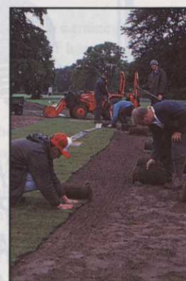
Laying the Rolawn 'Advantage' turf
