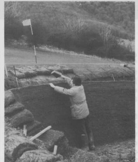
Final rows of turf laid. Edges were stepped down to allow for shaping.
