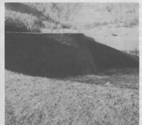
The completed job!
