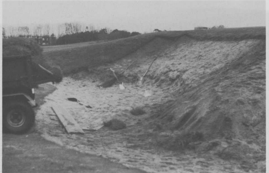
Old turf stripped from original bunker face in preparation.
