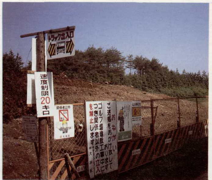
'Communications' to lorry drivers bringing material.
