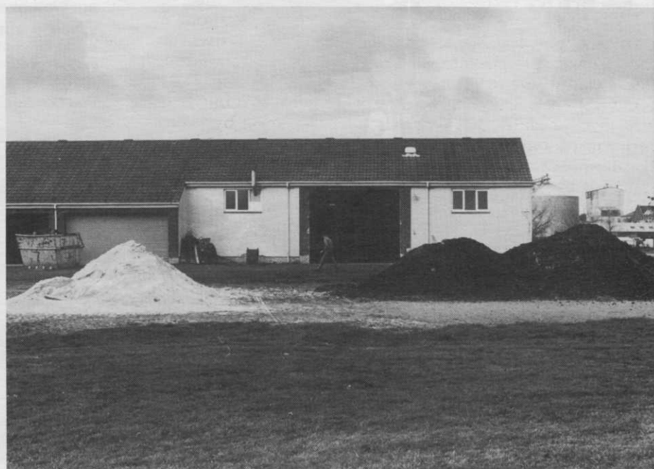
Expansive equipment sheds.
