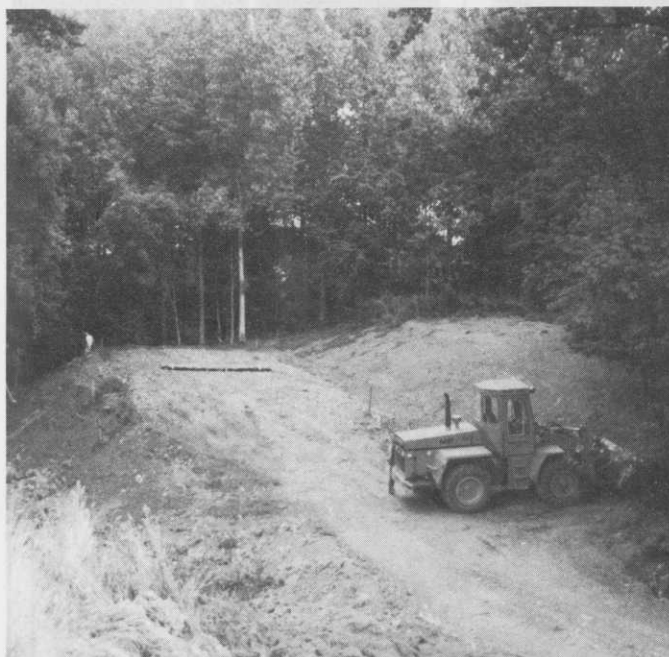
Ground work at Cherwell Edge.
