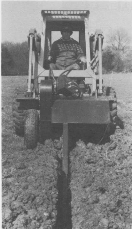
The Skid-Steer Trencher.
