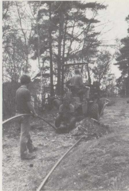
Pulling in the pipe work.
