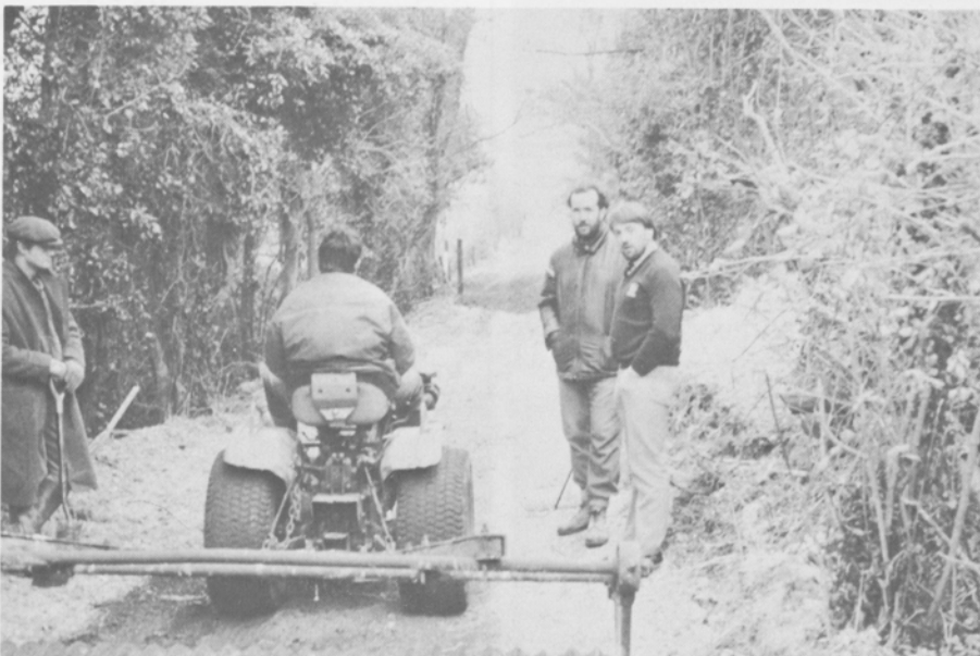
Resurfacing work to a public bridle path...
