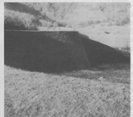
The completed job!
