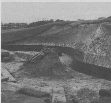
Several rows of turf laid in early stages of construction.
