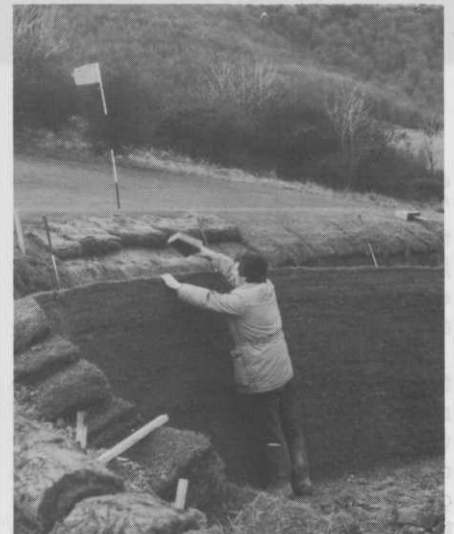
Final rows of turf laid. Edges were stepped down to allow for shaping.
