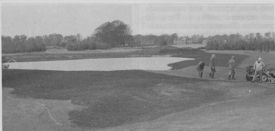
Greenstaff constructed this impressive lake.
