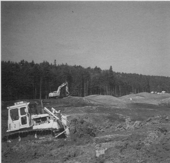
Heavy machinery contouring fairways.
