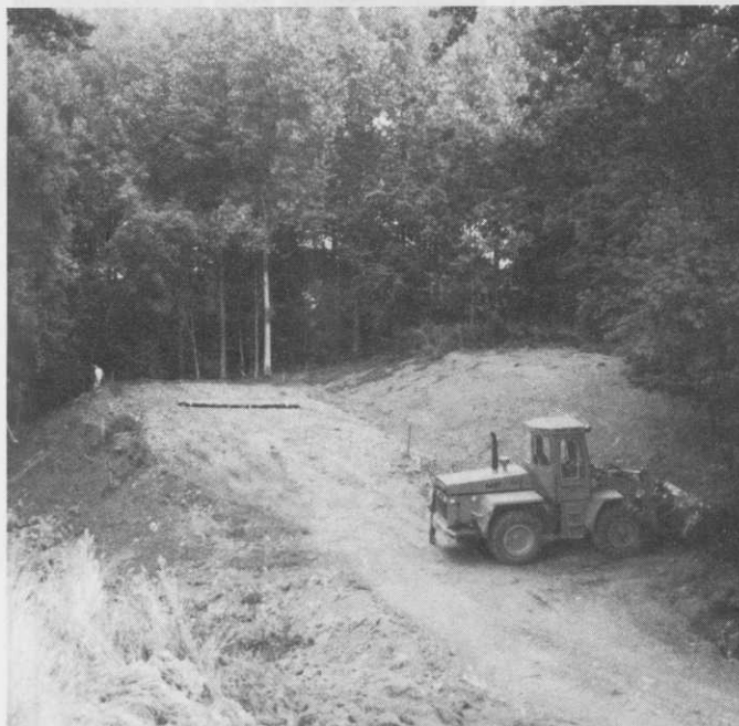
Ground work at Cherwell Edge.
