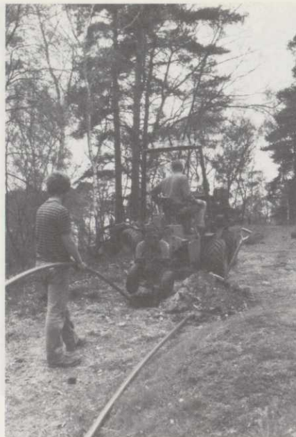
Pulling in the pipe work.
