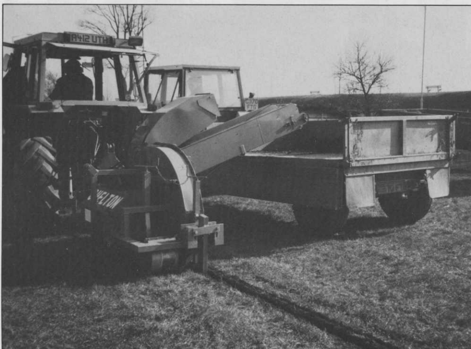
A tractor operated supertrencher cuts a 2" wide trench. The excavated soil can be used on other parts of the course
