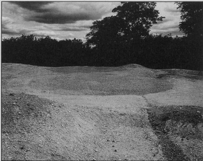
Early stage of construction to the 2nd green, showing the stone base.
