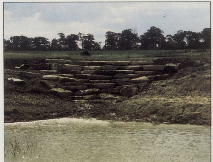
Waterfall built by the M.S.C. labour linking the two lakes.
