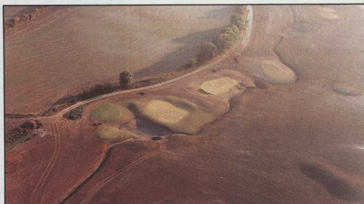
Aerial view of the 1st and 11th holes including lake and feed ditch at the recently completed Graveley Golf Course near Stevenage
