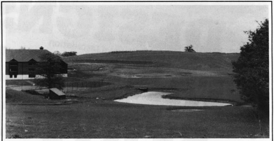
18th green and lake constructed at Botley Golf and Country Club
