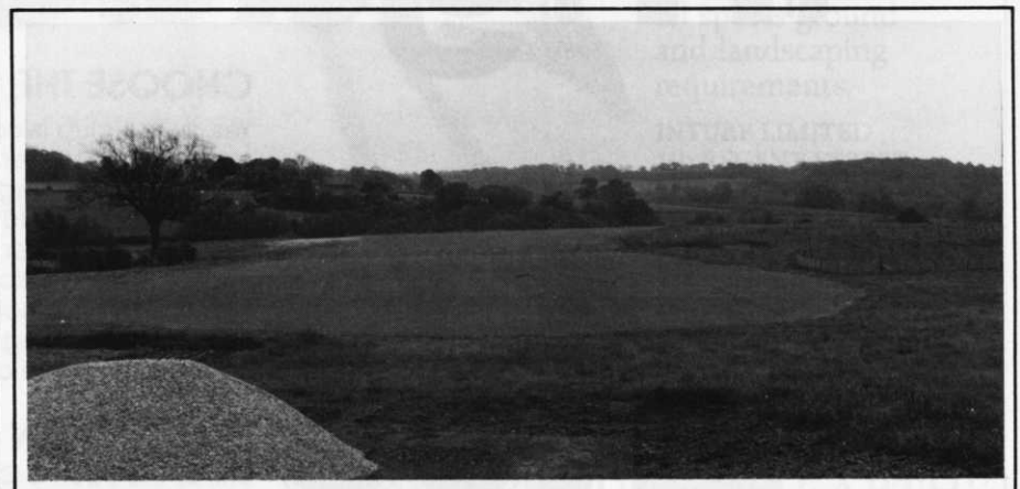
Tee and fairway construction at Botley Golf and Country Club
