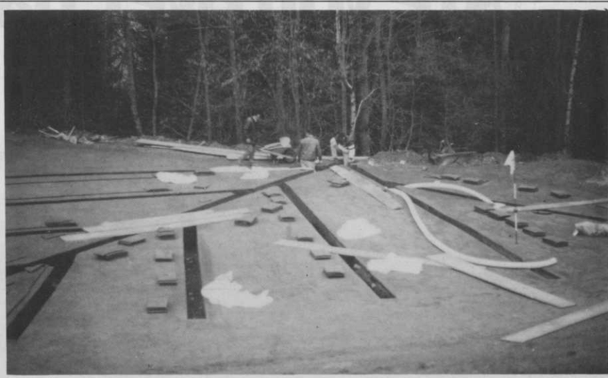
Complete new drainage system of green 12
