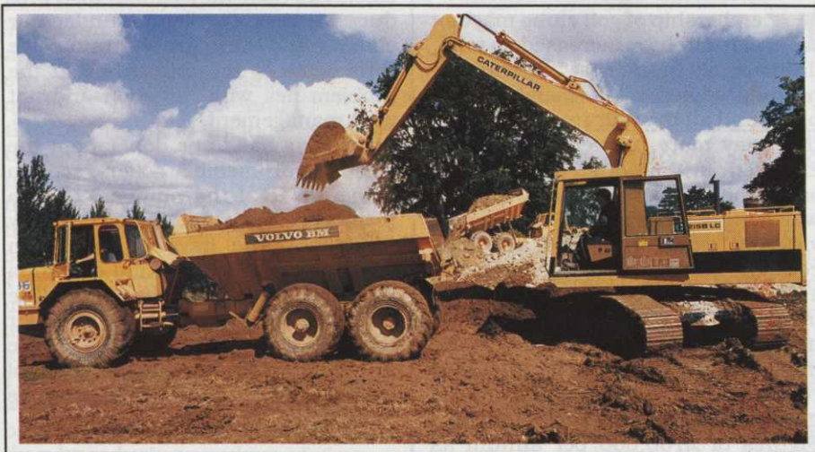
The use of special plant and good materials are essential
