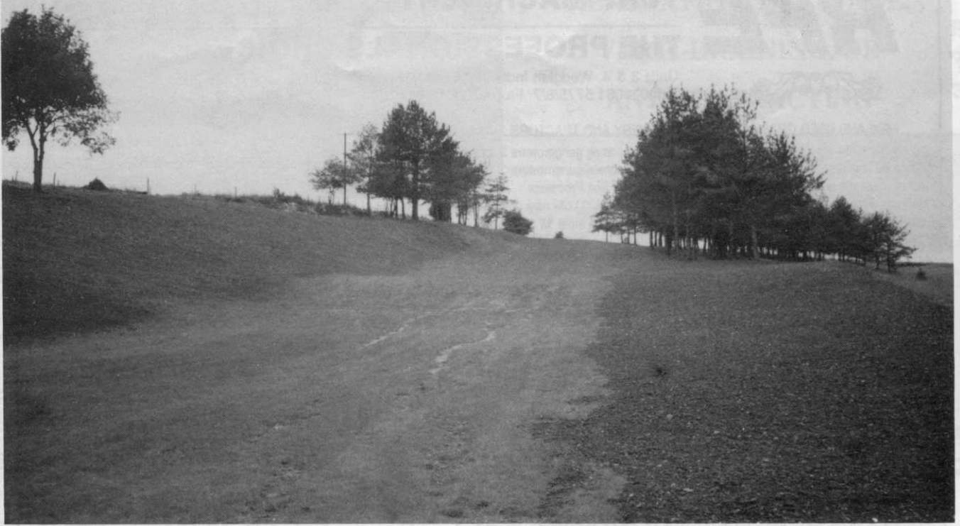
View of fairway from a tee shot landing spot. The position marked by small bush on horizon between gap in the trees. Exposed soil left and right is where features were modified this autumn to enlarge playing surface width.
