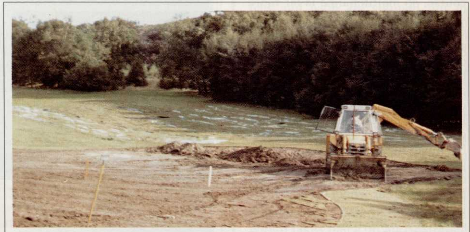
Excavation starts on the fifth green. Lifted turf laid out on polythene sheeting on edge of the fairway.
