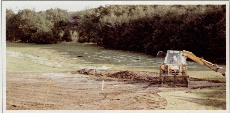
Excavation starts on the fifth green. Lifted turf laid out on polythene sheeting on edge of the fairway.
