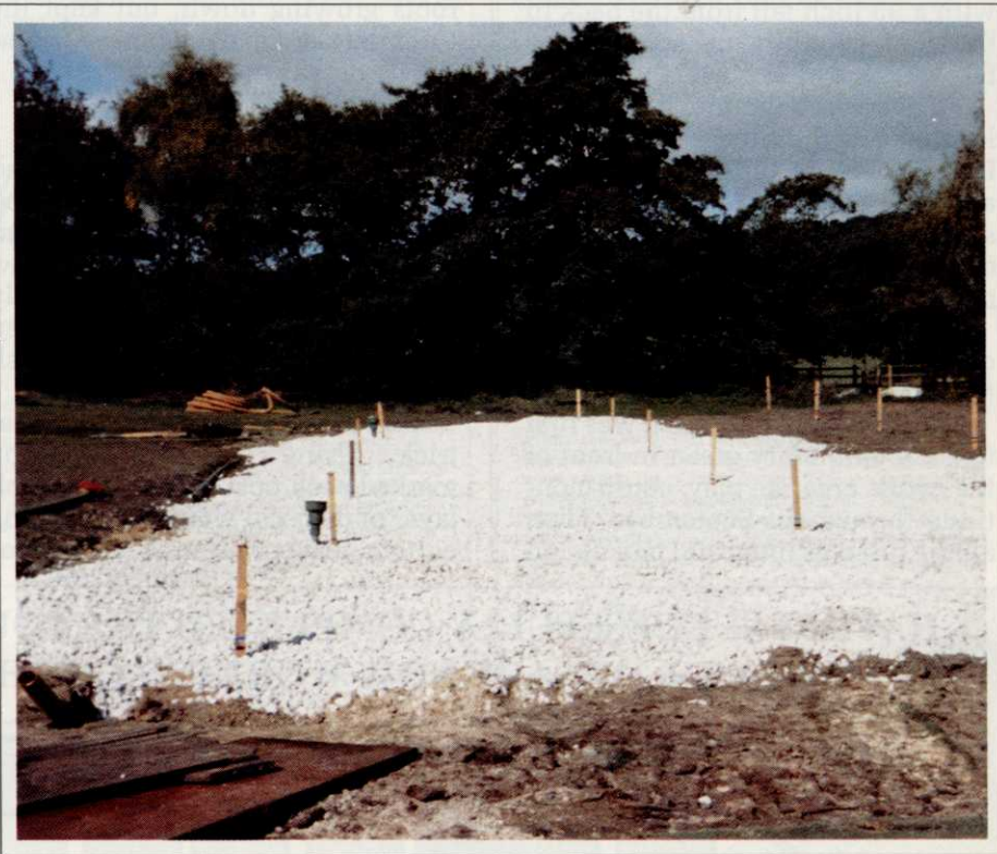
Hard limestone used in the re-construction of the fifth green at Shipley.
