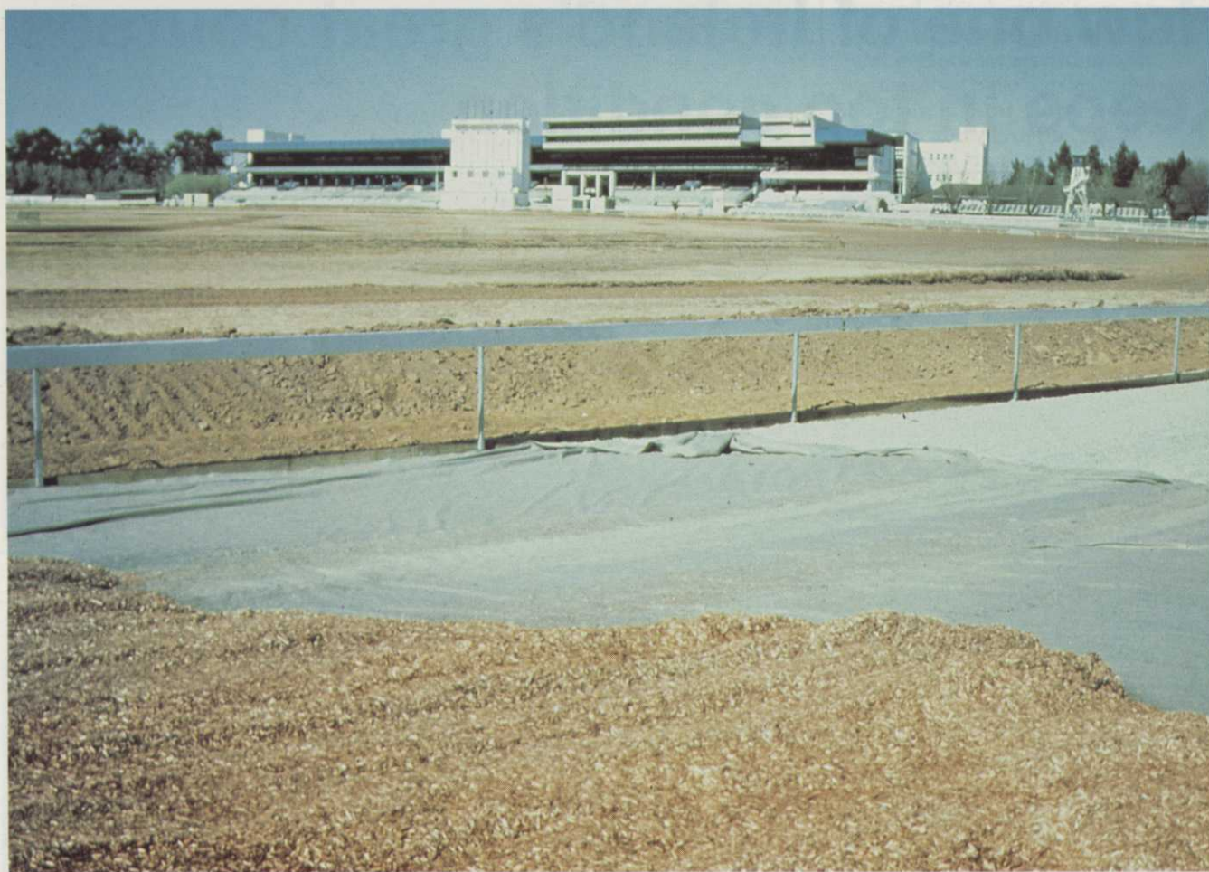
Geotextiles being used in the construction of a sports ground
