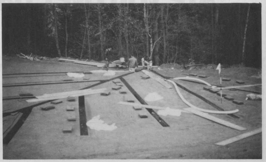
Complete new drainage system of green 12
