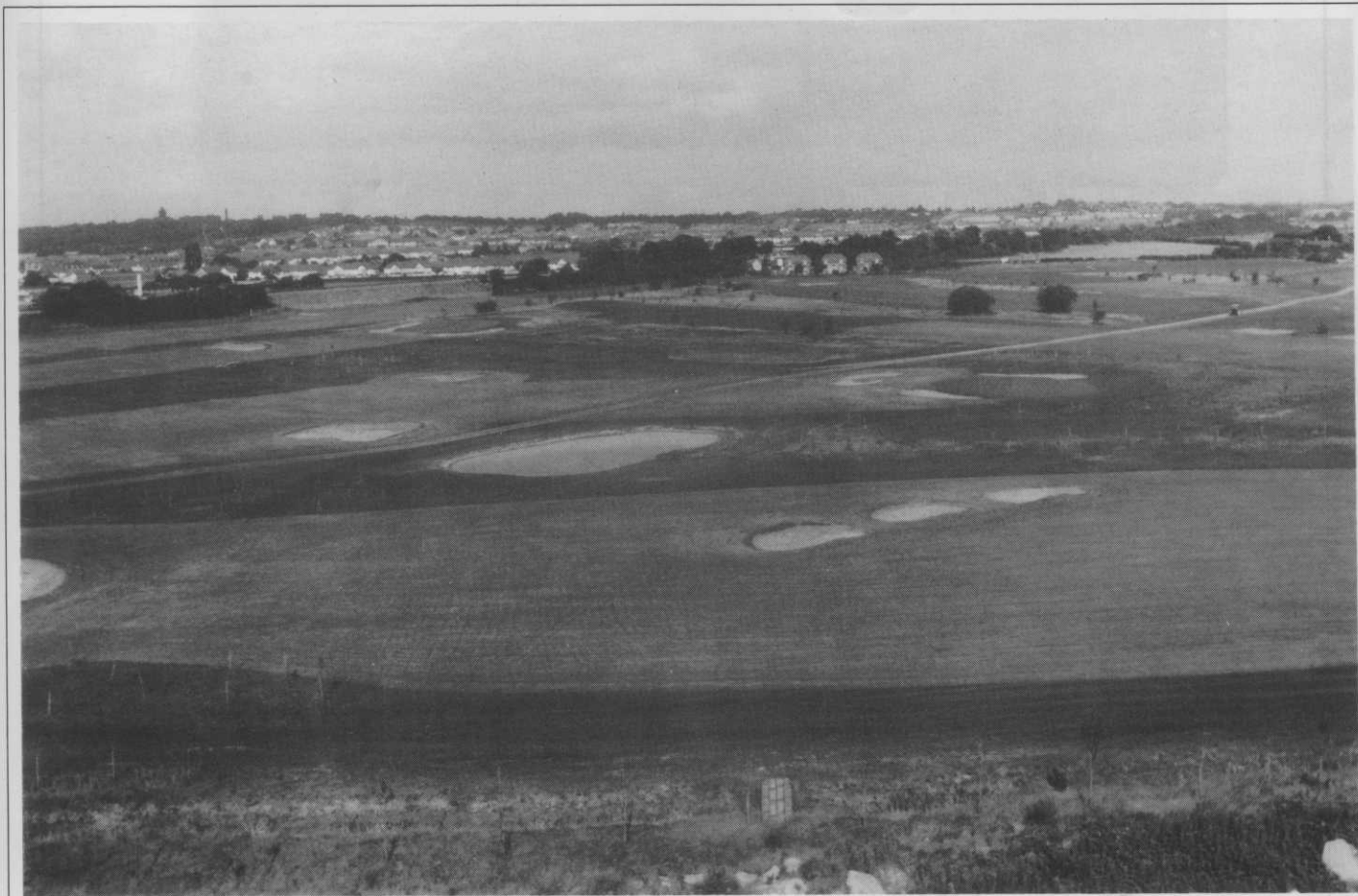
Fairlop Waters Golf Course where formidable drainage problems had to be overcome before construction could begin.
