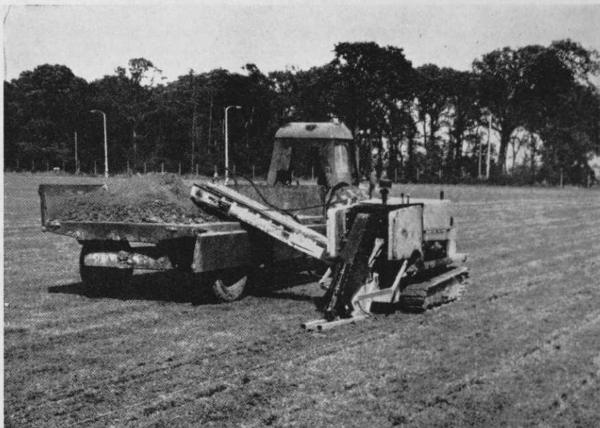
Davis Trencher supplied by L. D. Bourgein (Oxford) Ltd.
