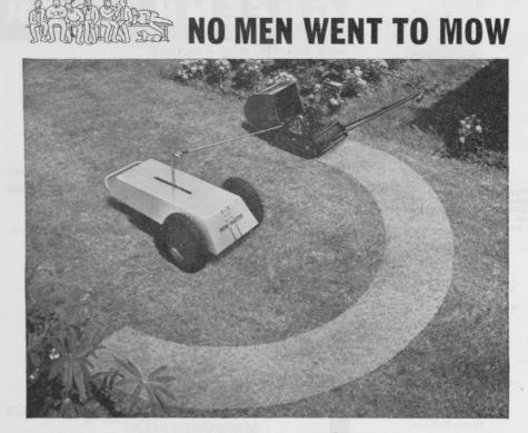
The Remploy MOW-MASTER takes the place of the man in charge of the motor mower and leaves him free to do other jobs. The MOW-MASTER is something *entirely new* to ground keeping. It is the first fully automatic mower attachment at a low cost.
