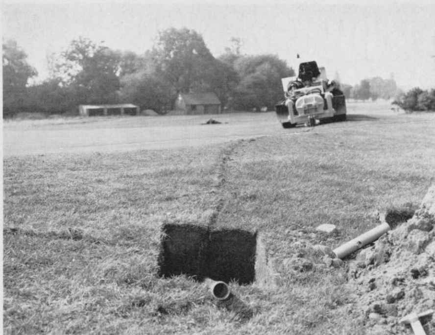
Mole ploughing supply pipe around a green. Note the negligible disturbance of the turf. Photograph: Wright Rain Limited
