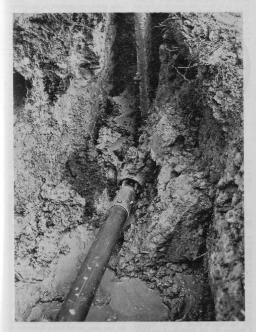
Laying Chemidus 3000 uP.V.C. 3 ins. pipe by mole plough in heavy Oxford clay for the West Wilts. Water Board at Wincanton recently. The 3 ins. Chemidus pipe is attached to the 6 ins. expander by means of a collar adaptor. The mole plough blade was set at a depth of 3 ft., and a 200 yd. length of plastic pipe was drawn underground from a prepared entrance. The blade of the mole plough can be seen at the top of the picture.
