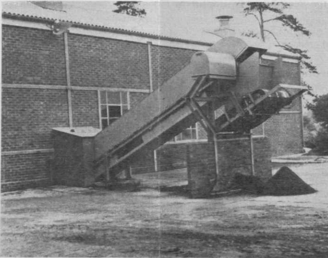
The compost conveyor and glass extractor.
