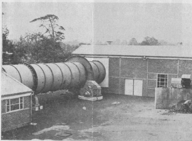
The "Dano" stabilizer and screening building.
