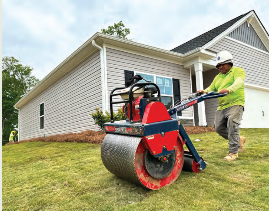
Installation crews at Saluda Hill use hydraulic, self-propelled rollers for sod installation.
