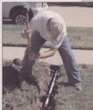
Hammer Sidewalk Sleever & pipe under obstacle
