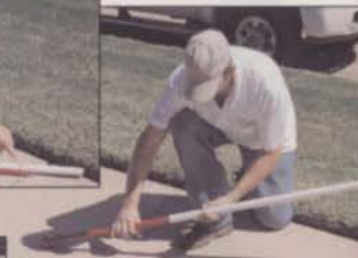
Place Sidewalk Sleever inside pipe
