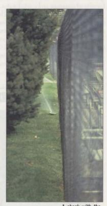
A check with the landscape plans while designing the system would have indicated that rotor heads were the wrong choice for this area.
