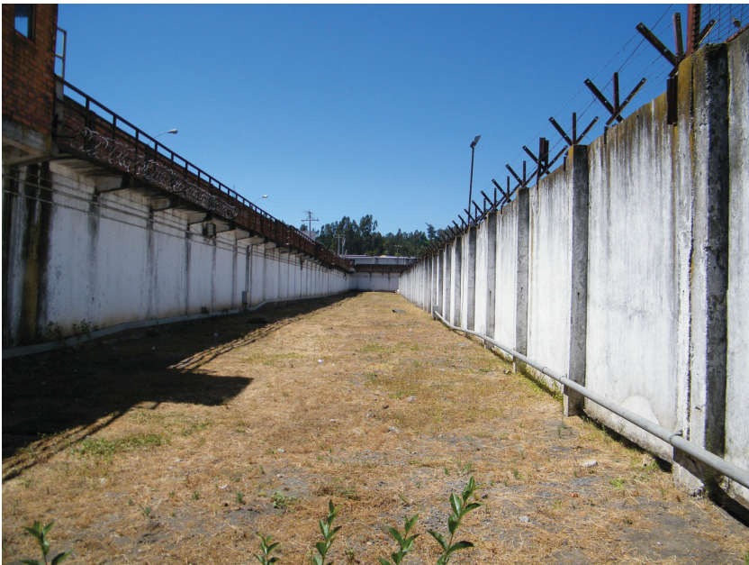
Figure 8.14 Double-walled security area with guard towers in Concepcion prison, Chile
