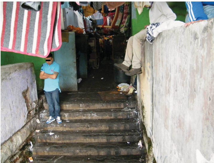
Figure 8.12 Inadequate hygienic and sanitary conditions in an overcrowded traditional Chilean prison. Entrance to a prison block. CDP-Santiago Sur prison, Chile
