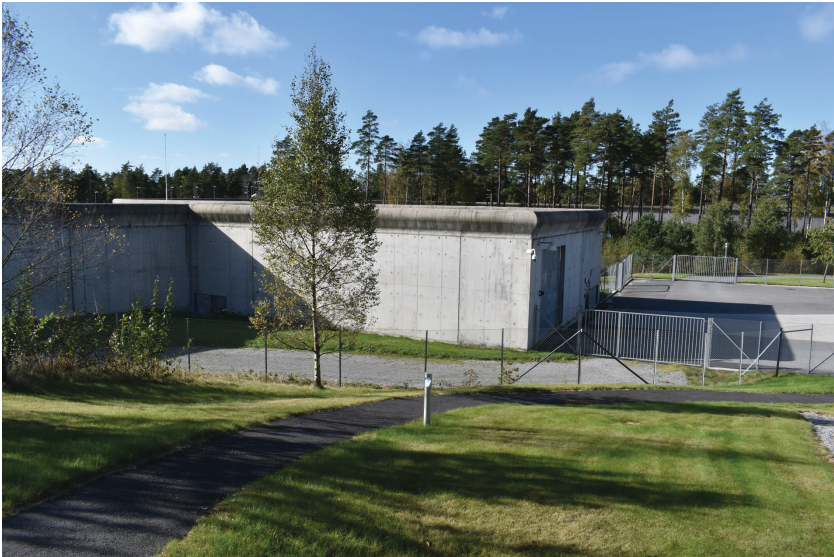
Figure 10.32 Halden Prison, Norway, perimeter wall
