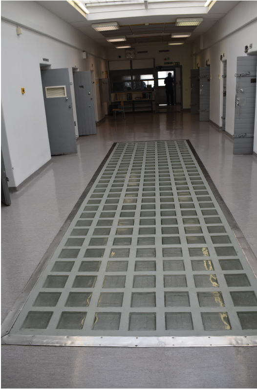
Figure 10.7 Helsinki Prison, Finland. Overhead lighting with daylight using skylight and lighting of the lower floor through the glazed floor
