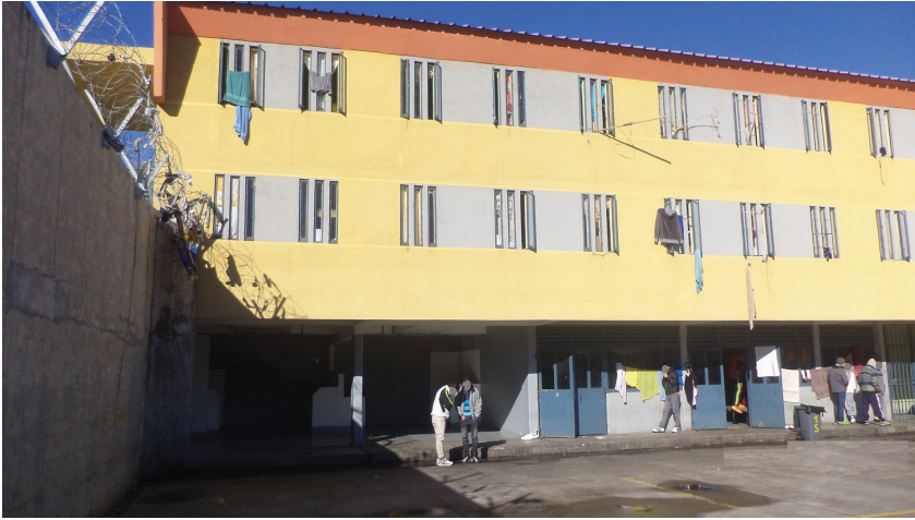
Figure 8.6 Inmates' block yard at Bío-Bío prison, Chile (PPP Contract)
