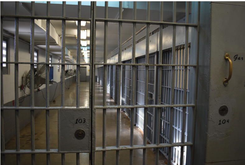
Figure 9.13 Louisiana State prison “Angola” Camp B. Row of cells (right) separated from the windows by a corridor, to provide daylight (left)
