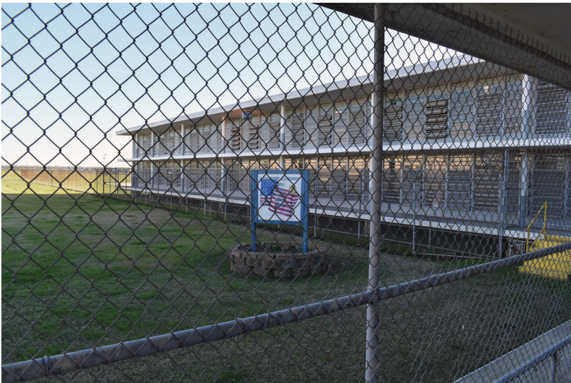
Figure 9.15 Louisiana State prison “Angola” Camp A. View from the exterior façade of translucent polycarbonate windows
