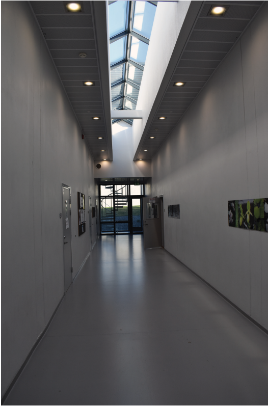
Figure 10.8 Skylight using daylight. Educational area Halden Prison, Norway
