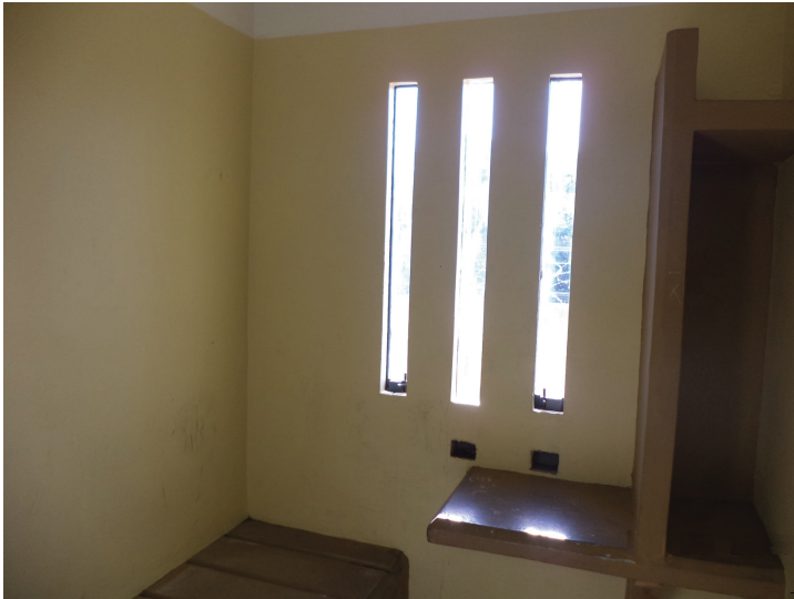
Figure 8.9 Narrow prison cell windows – PPP Bío-Bío prison, Chile
