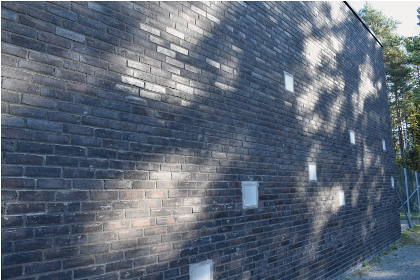
Figure 10.11 Soft daylight through walls (outside view of the prison chapel). Halden Prison, Norway
