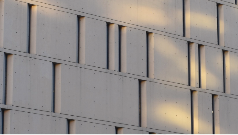
Figure 9.12 Close up of windows at Chicago Metropolitan Correctional Center
