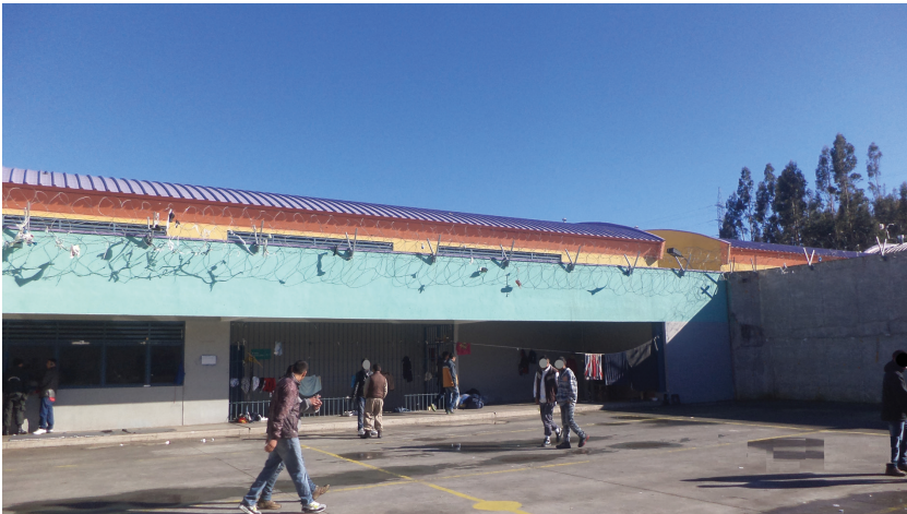
Figure 8.7 Block's workshop area, at Bío-Bío prison, Chile (PPP Contract)
