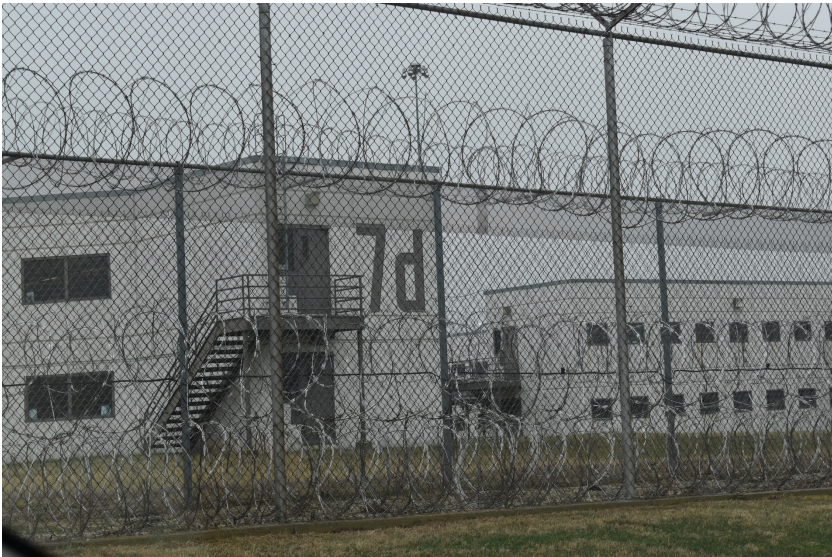
Figure 9.7 External fence area, Luther Lockett Correctional Complex, Kentucky
