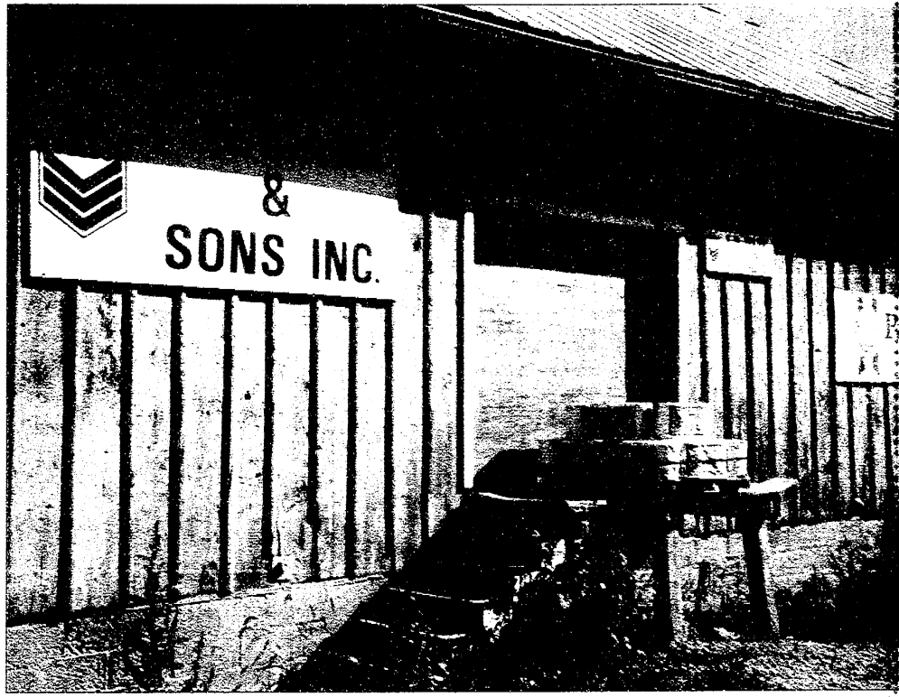
This building on Boettner Road is likely the oldest of the several that comprised the E.G. Mann and Sons feed mill that closed on Sept. 30. Up until that time, all signs (right) indicated that the business could fill a variety of needs for local farmers.
