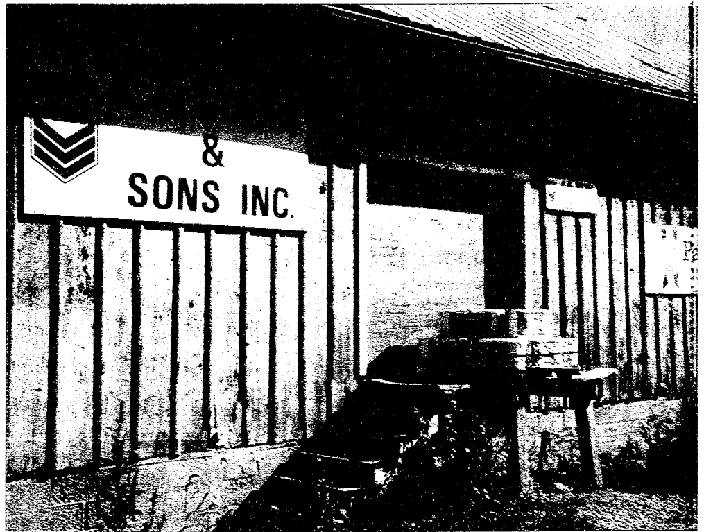
This building on Boettner Road is likely the oldest of the several that comprised the E.G. Mann and Sons feed mill that closed on Sept. 30. Up until that time, all signs (right) indicated that the business could fill a variety of needs for local farmers.
