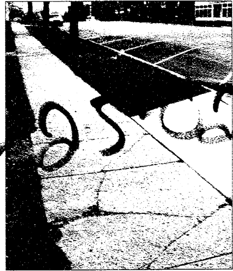
Sidewalks like this one will soon be replaced under a village program approved at last week's meeting.
